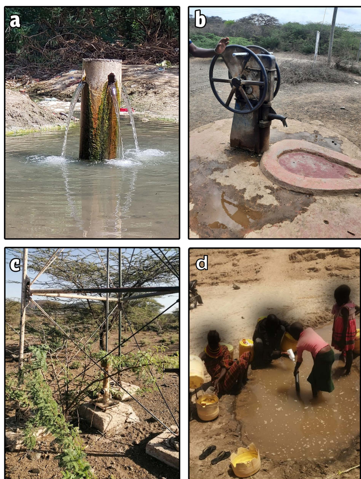
Fig 4. Boreholes abandoned due to: (A) poor water quality, (B–C) breakdown, (D) Turkana residents fetching water from a broken piped water supply.
